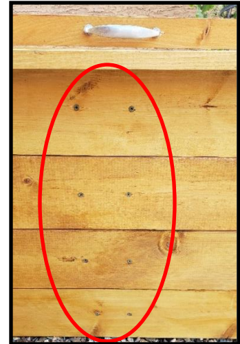
Screws securing 6" x 2'
